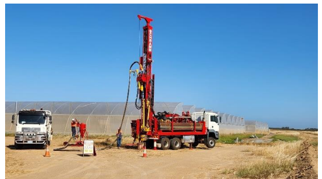
Drilling rig in action at Yamatji Fresh
